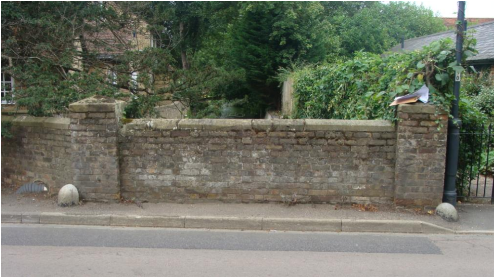
Picture 18 – Simply designed bridge over the River Mimram.
