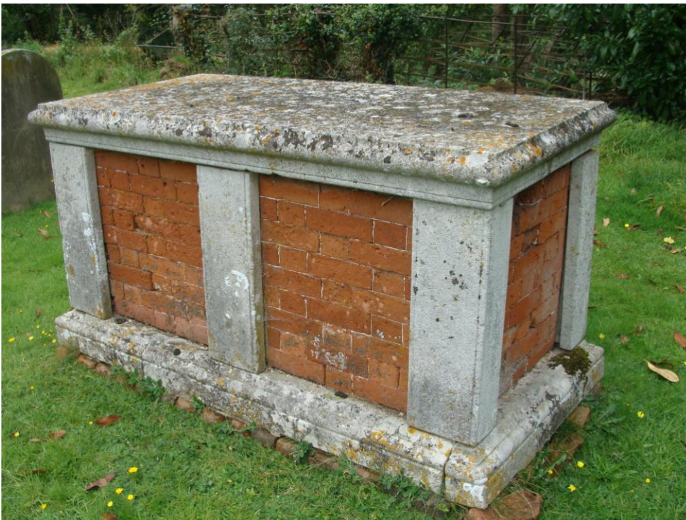
Picture 14 – One of many fine chest tombs in the churchyard, this one being of stone and rubbed brick.
